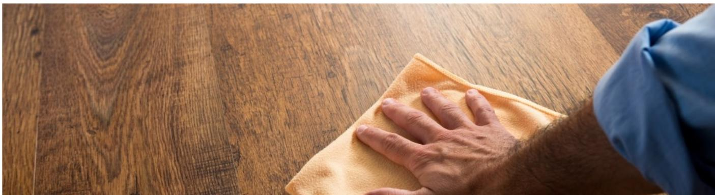
It is not recommended to use abrasive materials or aggressive chemicals. It is forbidden to use steam vacuum cleaner for cleaning waxed floor, since wax when getting hot may become liquid and it can be easily cleaned from the wood.
